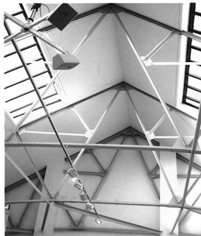
Millennium Court Arts Centre; roof girders Photo: Barbara Freeman
